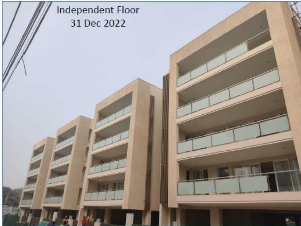
Internal Finishing in progress for Plot no W1A/5 to W1A/2
